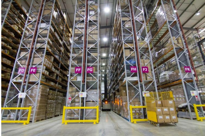
Investment in new purpose-built Components distribution centre
